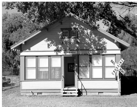
Railroad section house on the Skull Valley Historical Society grounds. Learn the history of it..
